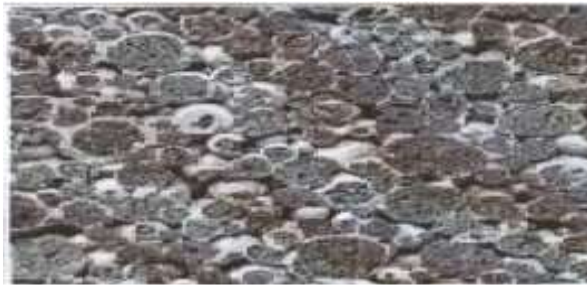
Figure 2: Lightweight aggregate concrete
