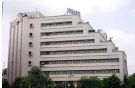
Fig 08 Vertical Geometric Irregularity
