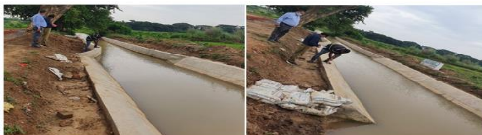
Fig. 9 Rebound hammer testing at canal lining portion on 28 days of maturation
