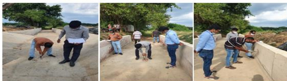
Fig. 8 Rebound hammer testing at canal lining portion on 14 days of maturation
