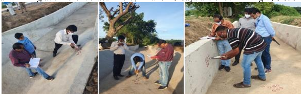
Fig. 7 Rebound hammer testing at canal lining portion on 7 days of maturation
