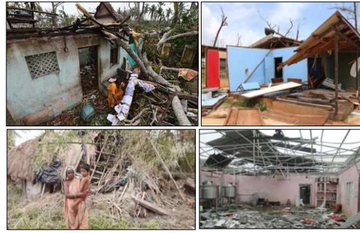
Figure 1.1 Destructions of buildings due to different cyclones
