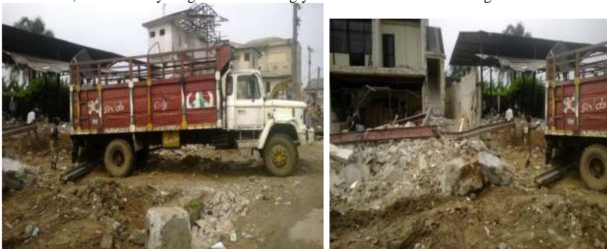
Figure 1: Demolition waste and transportation of demolition waste
