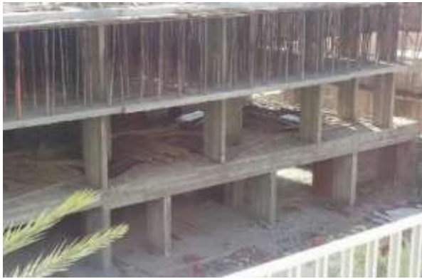
Figure 2:- Transfer slab With Column
