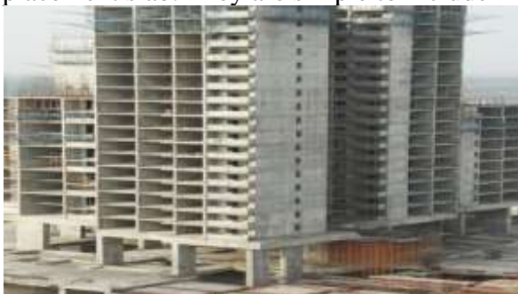
Figure 1:- Transfer slab With Shear wall
