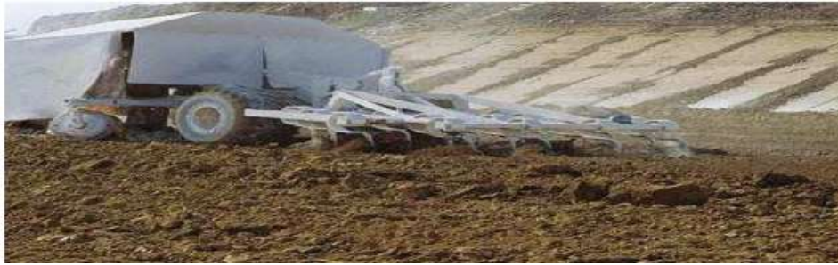
Figure 1: Shows the scarification of lime over the soil layer
