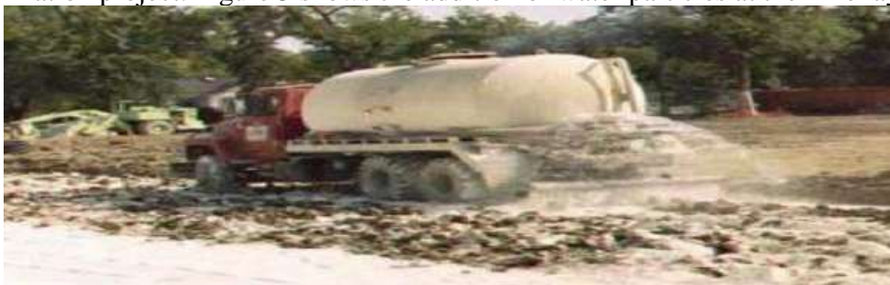
Figure 3 shows the addition of water particles at the lime layer
