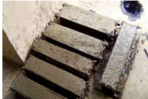
Fig.8 Casted of beams
