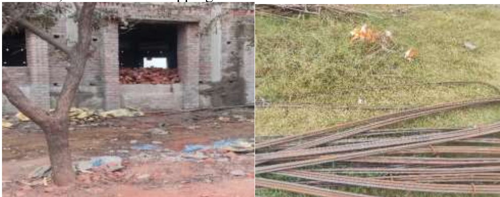
Fig(a) Improper storage of materials
