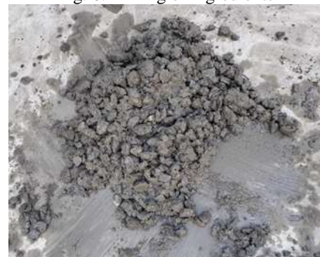
Fig. 7: Mixing of Concrete
