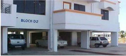
Figure 1: Open Ground Storey
