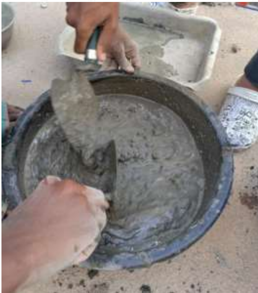
Figure. 7: Mixing of SCC
