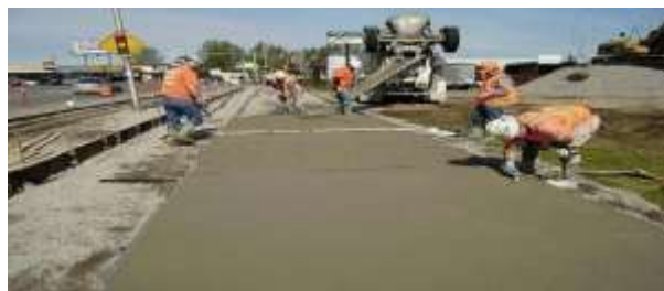
Fig 1. Road Grading construction
