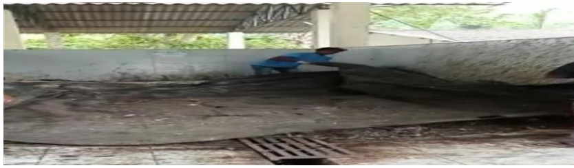
Fig3.4 Set up covered with Tarp
