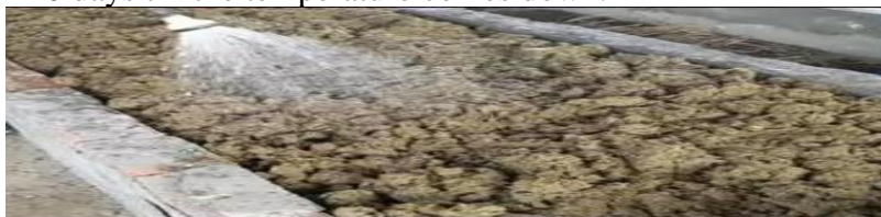
Figure3.9 Sprinkling of water
