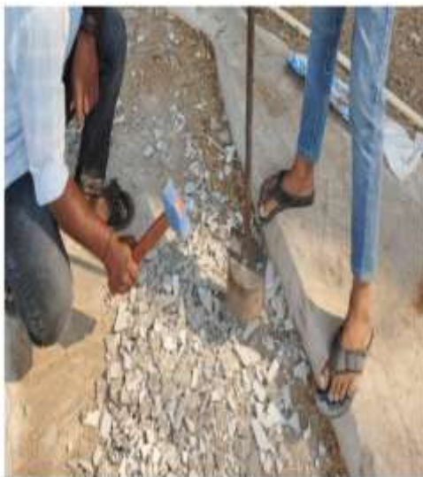
Figure .3 Crushing of tile waste by manual process.
