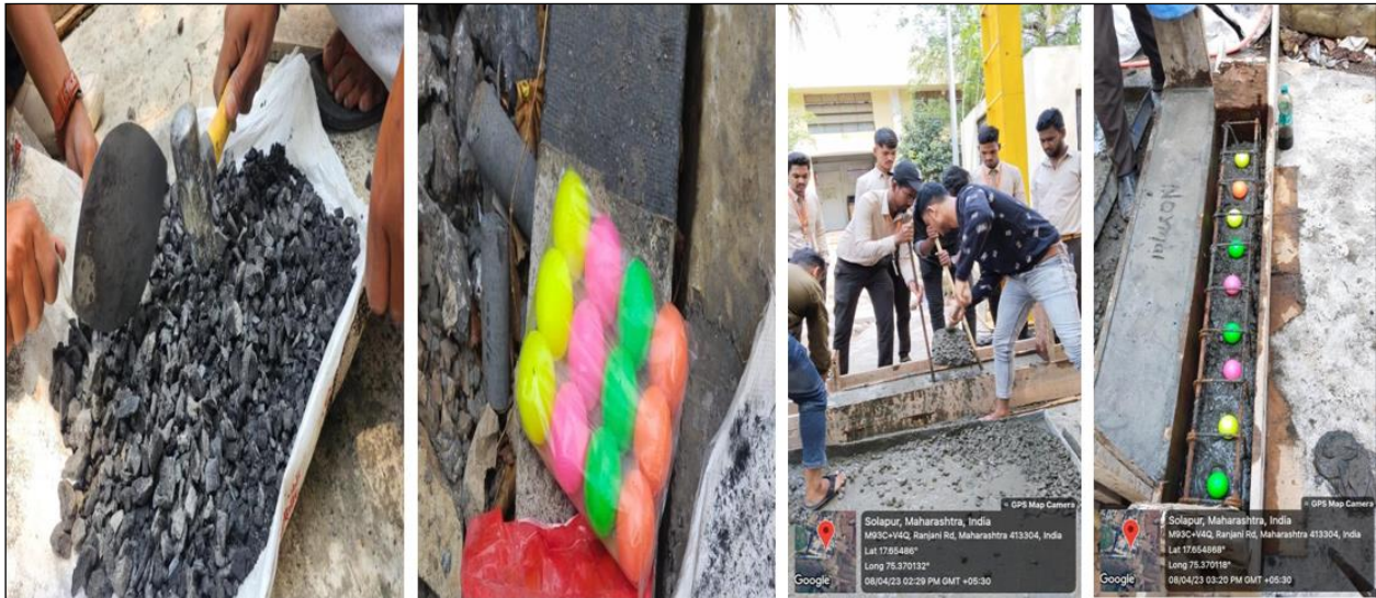
Figure 3 Coal for Mixing in concrete as reinforced material and Bubble for concrete making
