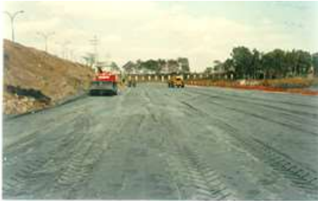
Fig 1: Compaction of fly ash with cement
