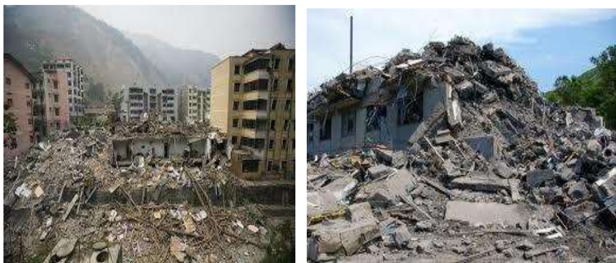
Figure 1-2&3: Hill Buildings Failure in Sichuan and Haiti Earthquake
