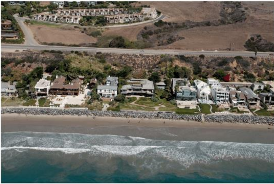
Figure 1- Rip-rap revetment armoring a section of the Malibu, California (USA) shoreline
