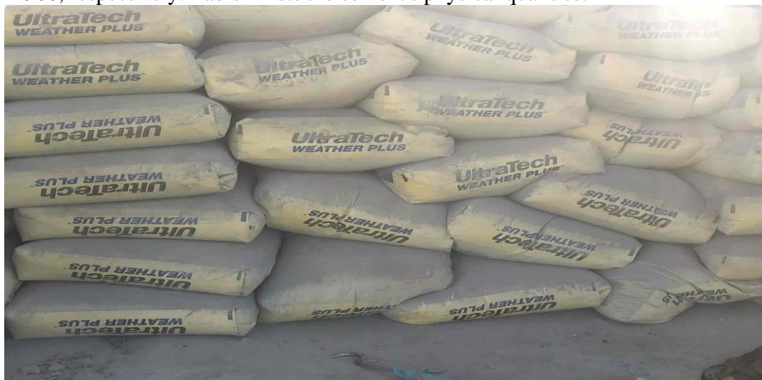
Figure 2 Stacking of Ultratech Cement in warehouse
