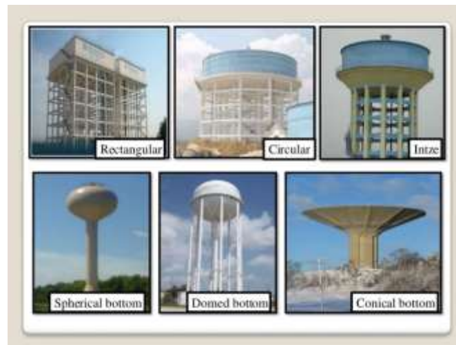
Figure 1: Types of water tanks
