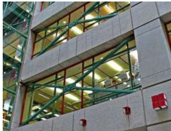
Fig.4 Friction Damper structure
