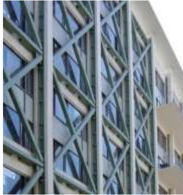
Fig.3 Steel Bracing Structure
