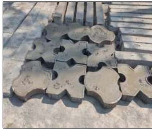
Fig – 3 –Setting of paver blocks
