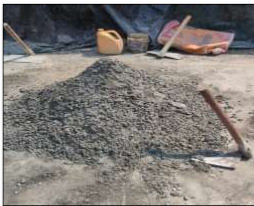
Fig – 2 – Mixing of Concrete Mix
