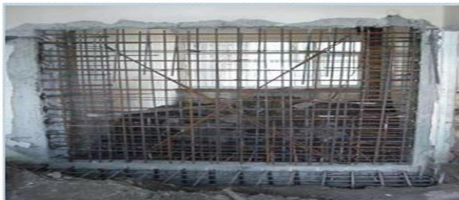
Figure 2- Additional shear wall
